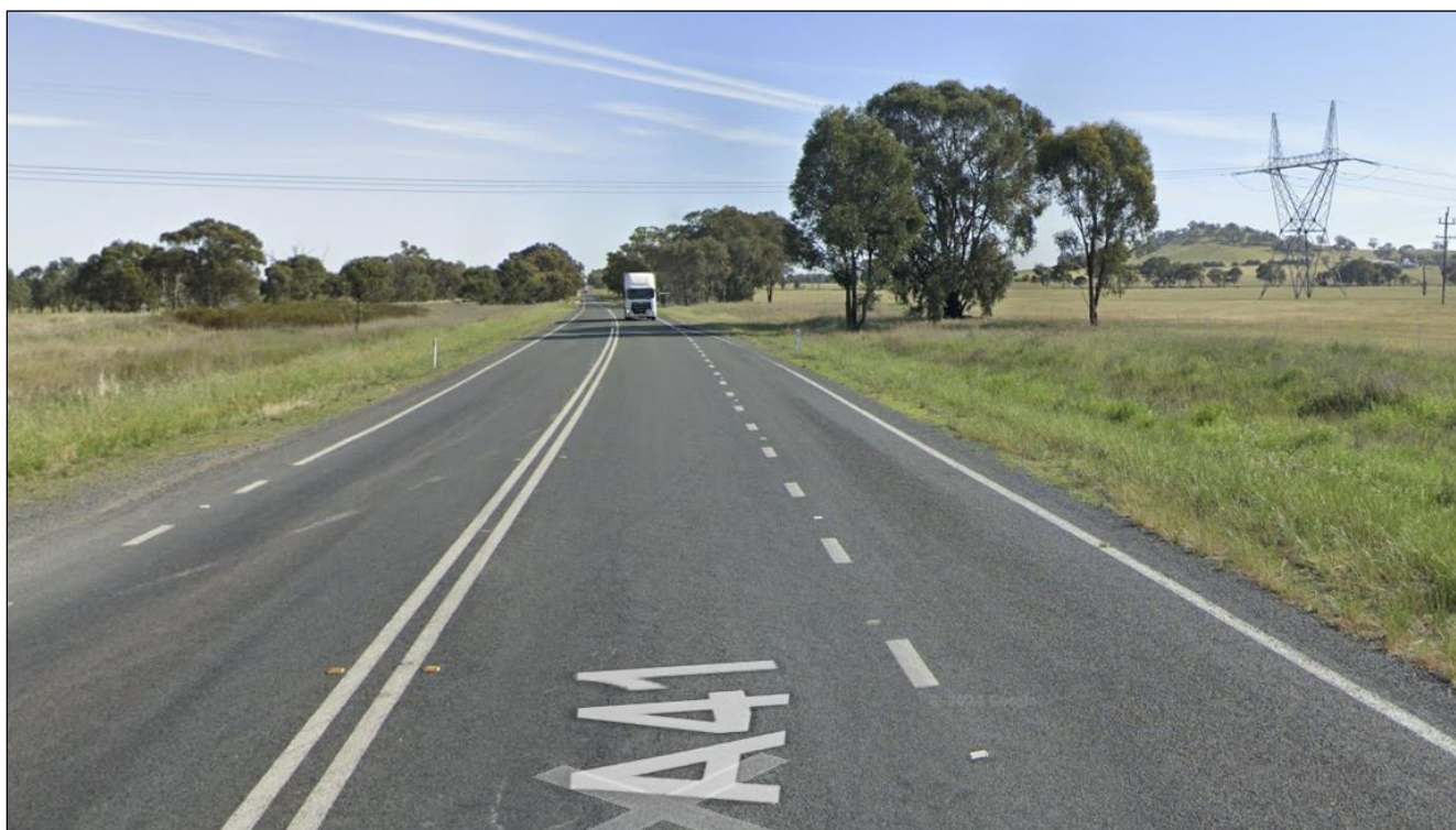
Figure 4: Olympic Highway – view north (source: Google Street View)
